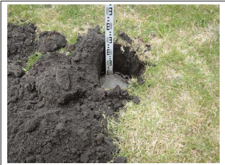
Test Hole 3 (Start)
